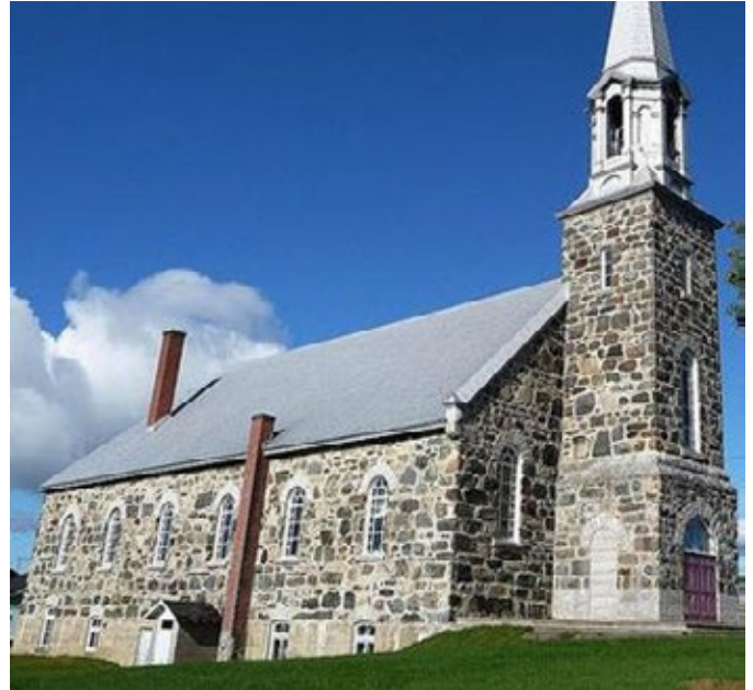
Turning a church in Saint-Alfred into a modern facility where food will be grown and stored
