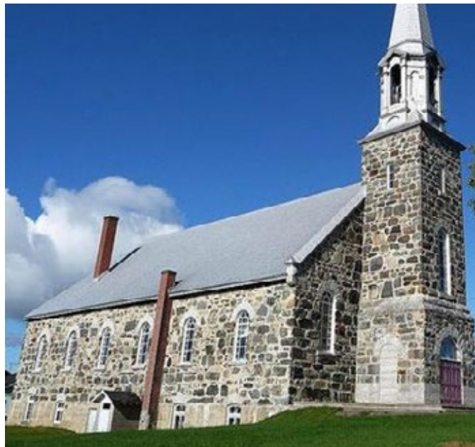
Turning a church in Saint-Alfred into a modern facility where food will be grown and stored
